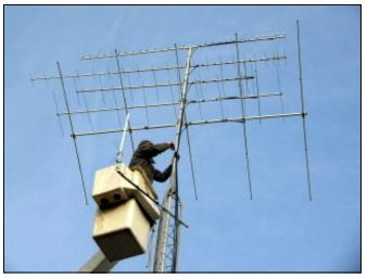
6 meter beam done. Lashing coax to mast
